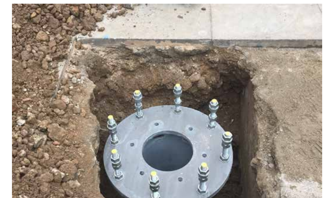
Pile cap with hold down bolts.
