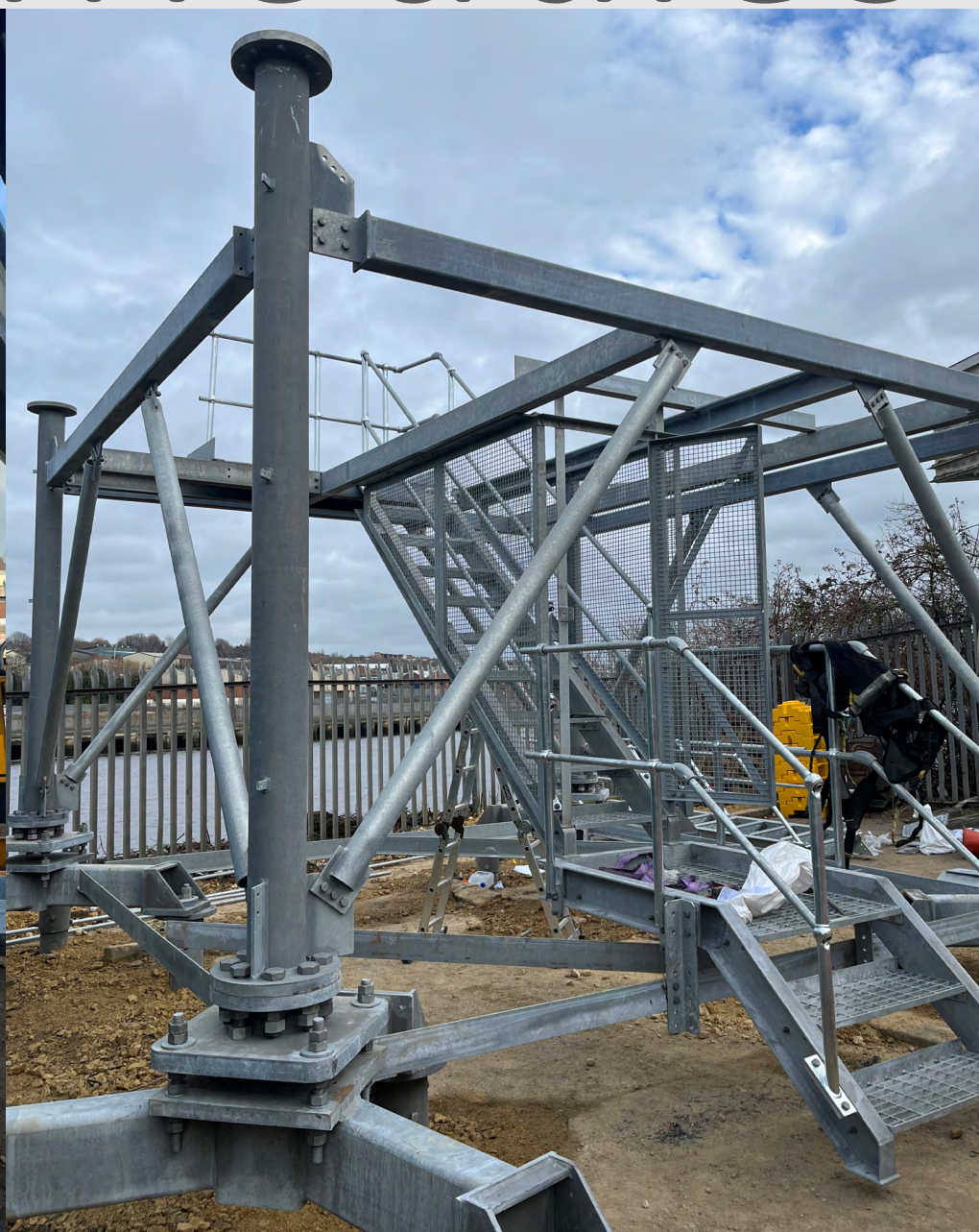
Internal staircase with security grill fitted to first tower module.
