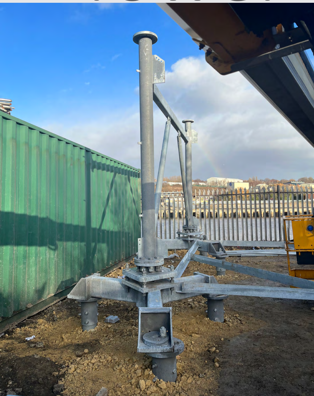
First tower section mounted on grillage.
