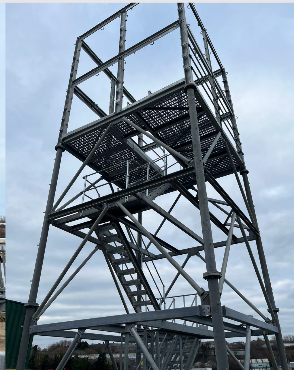
Full height of tower, with cabin frame.
