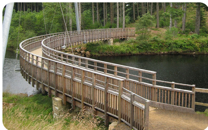
Lewisburn bridge at Kielder Forest inspired by The Elephant Bridge, with curved walkway.
