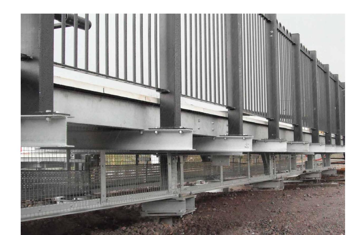
Fast installation with no concrete pour or curing time.
