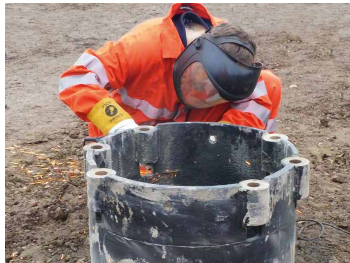
Cut pile to Height.
