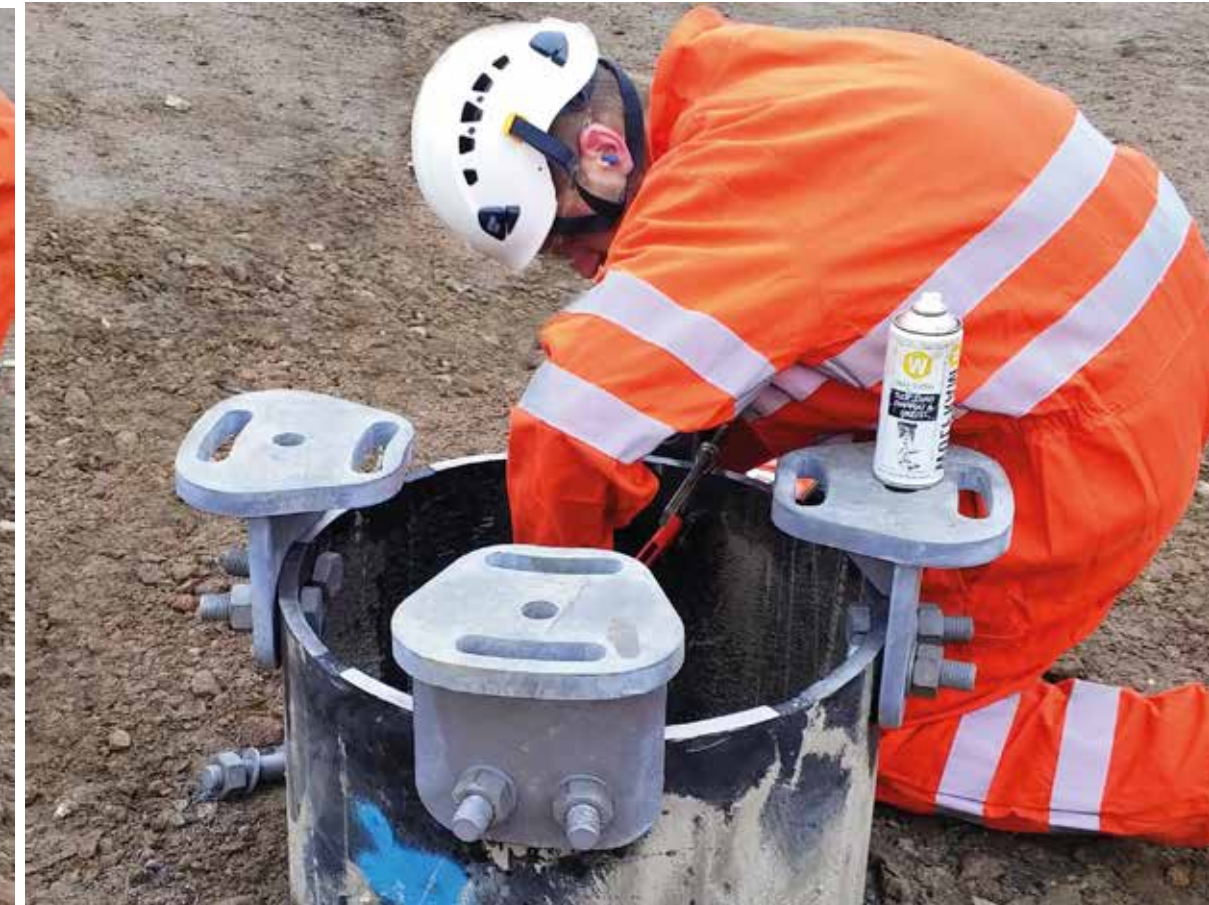
Bolt on Flexi-Pile Cap tabs.
