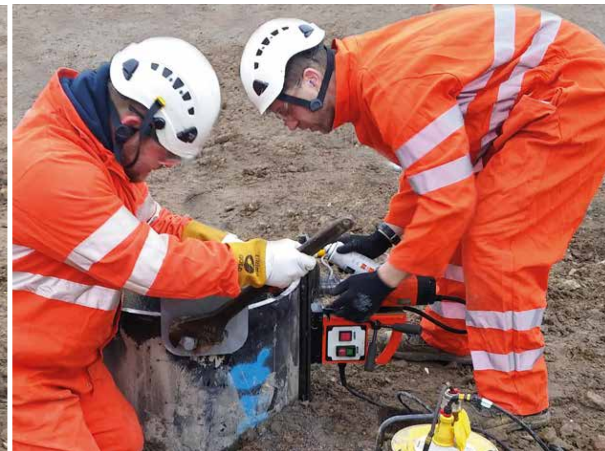
Drill holes using a template.
