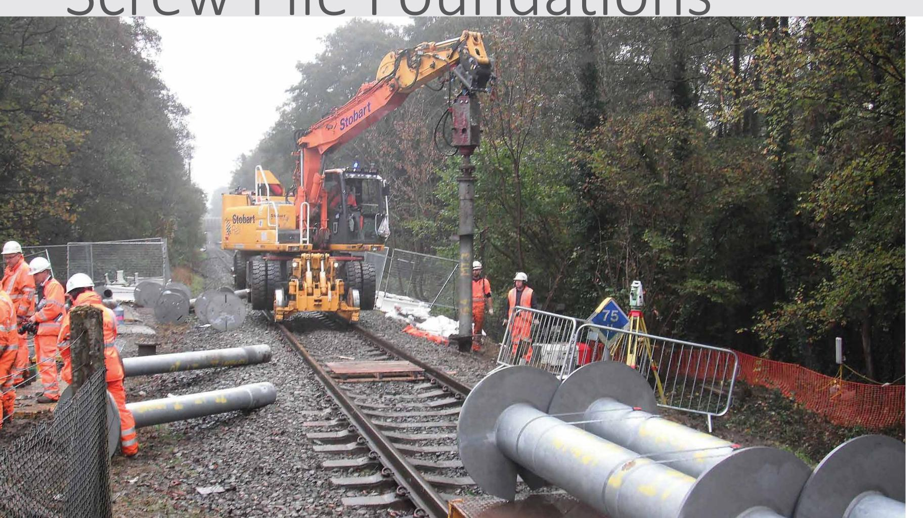
Screw pile & grillage foundations can be installed in a single shift, using a small team, torque motor and an RRV.
