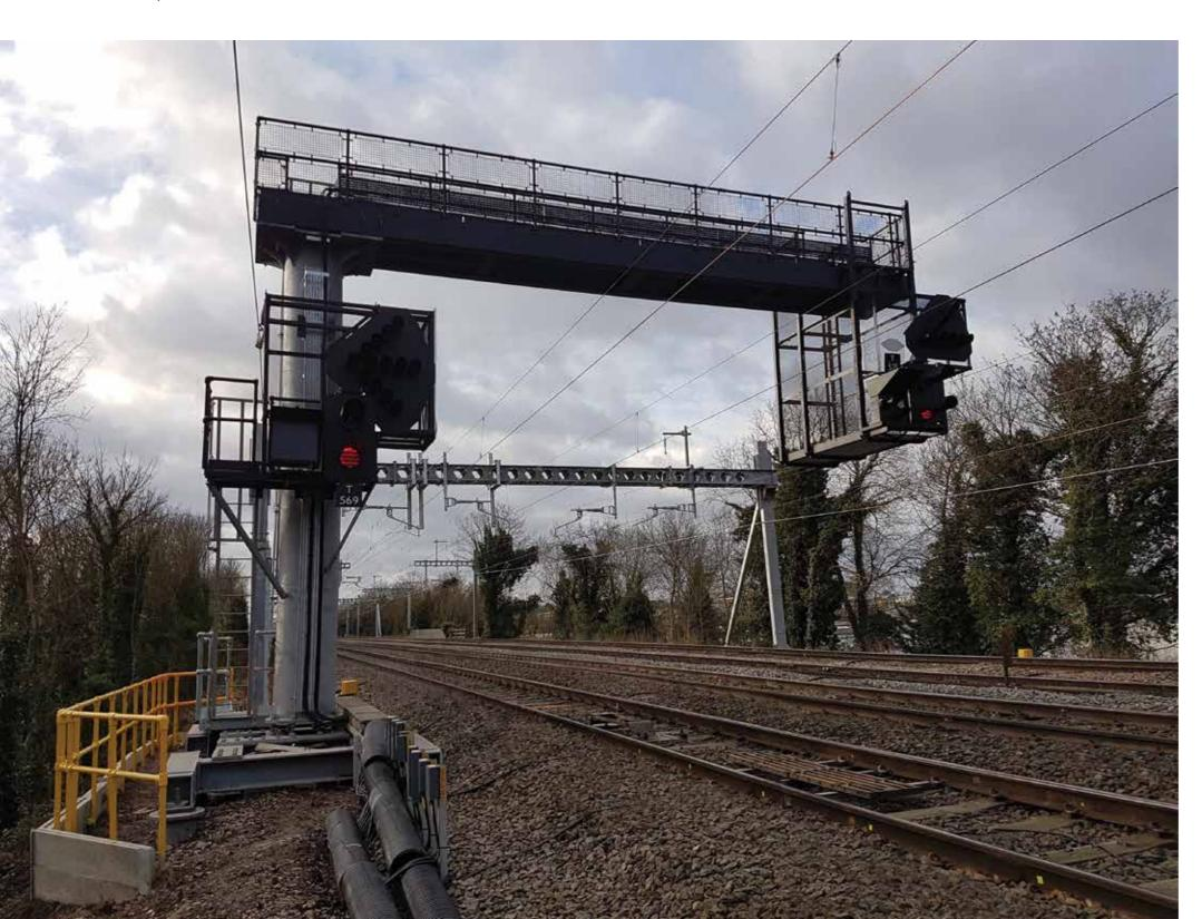
FLI Structures was contracted to design and manufacture a TTC with a span of 9m for Crossrail at Maidenhead. The structure incorporated a maintenance access walkway and access platforms. It supported two sets of signals, one in the dropper cage and one on the mast, all mounted on a rapid install FLI screw pile and grillage foundation.
