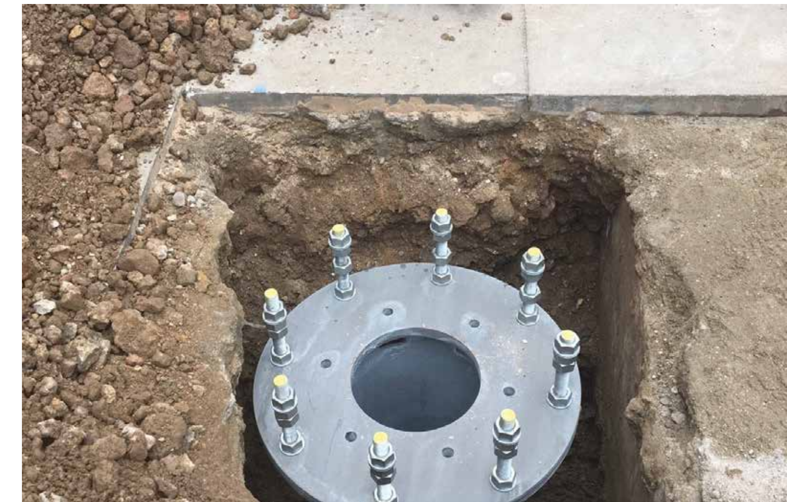
Pile cap with hold down bolts.
