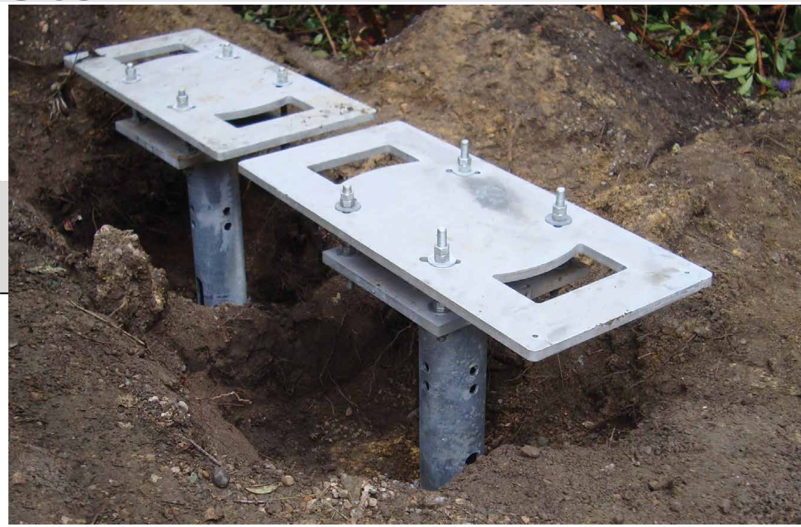
Cabinets mounted on single piles.
