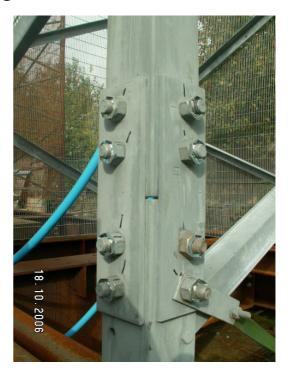
Fit the PAL nut onto the assembly and tighten using an open-ended spanner, until tight plus one half turn.
