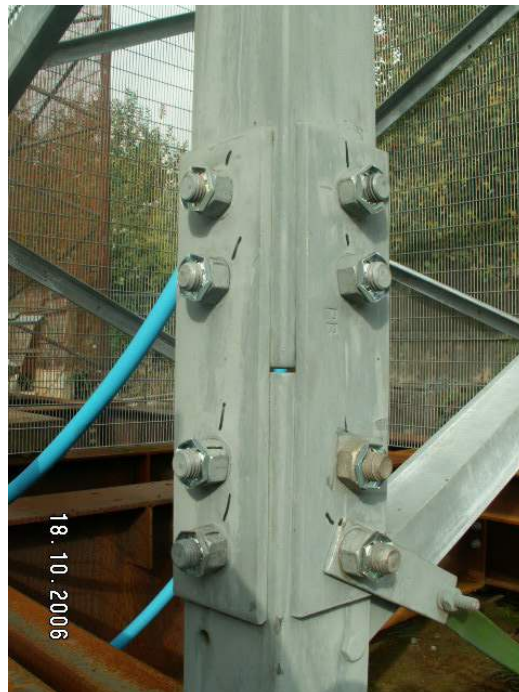
Figure 1 - Example of Match Marking
